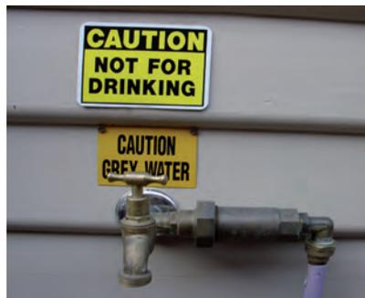
Below ground greywater treatment system. The Super Natural Grey unit was installed in the 12 unit Westswyck development in Melbourne by Sustainable Plumbing Solutions (top) Tanks (above) Greywater tap (left) Sink (below)
