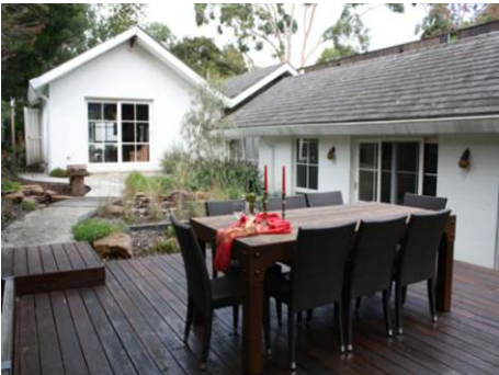
View across entertaining deck area
