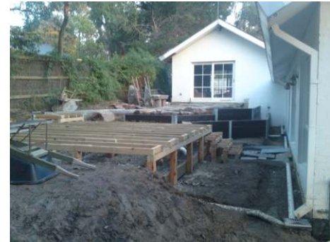
Deck construction and drainage
