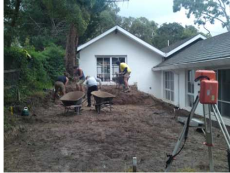
Excavation and grading
